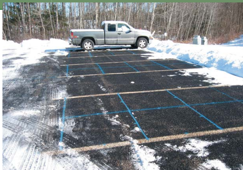
Figure 3. Comparison of dense-mix asphalt (left) and porous asphalt (right) on the same day, one hour after plowing.
