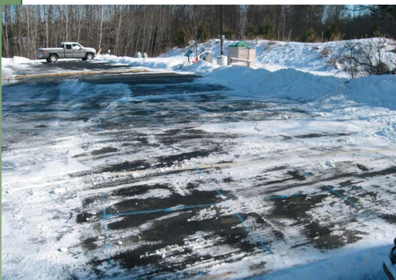
Figure 3. Comparison of dense-mix asphalt (left) and porous asphalt (right) on the same day, one hour after plowing.
