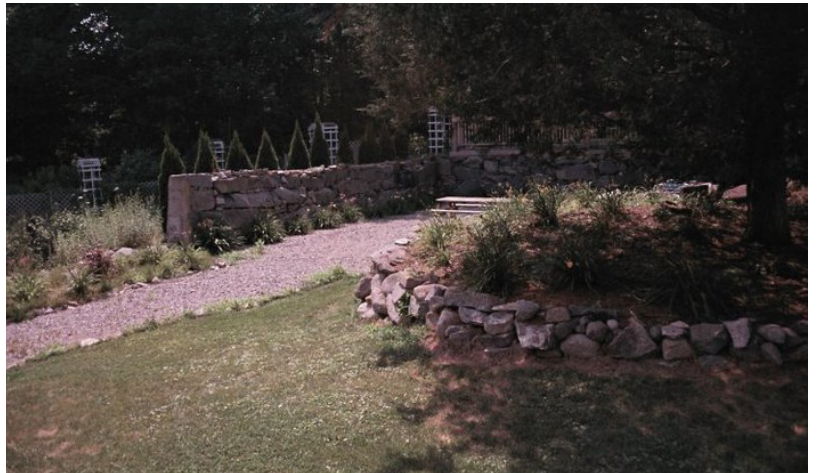
David Ripley's Newmarket barn renovation and original foundation
