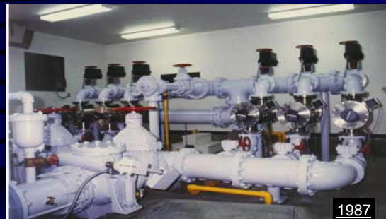
Aquionics MP UV for a PWS in Fort Benton, Montana
