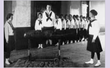
In 1915, New Hampshire College granted the Woman's League's request that women be permitted to use the gymnasium on the top floor of Thompson Hall each week.
