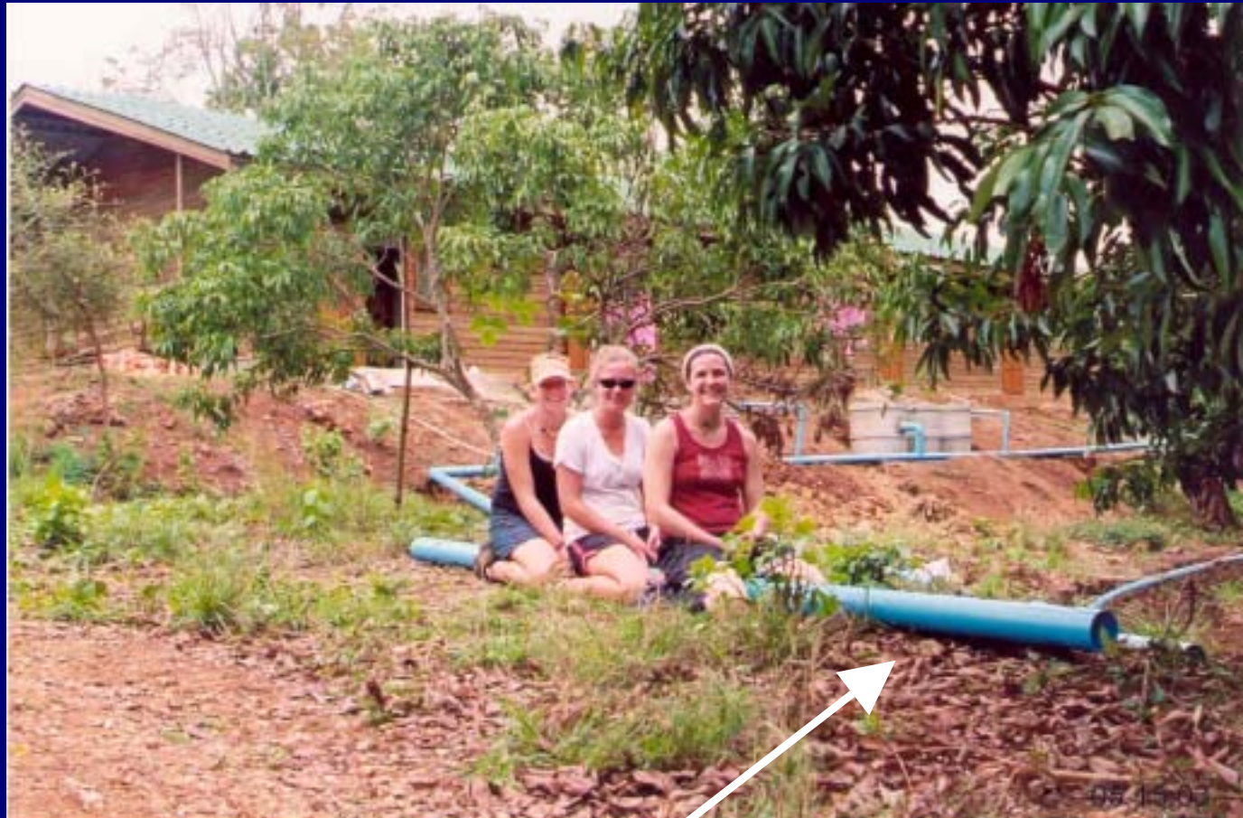
Piping the wastewater to the second leachfield
