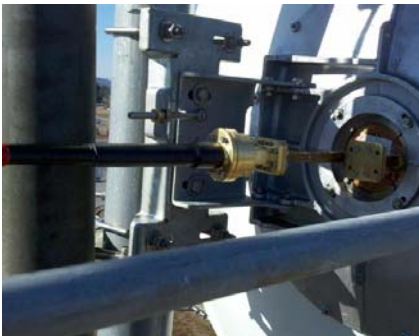
An unusual view: The back of a microwave dish installed on one of the towers.
