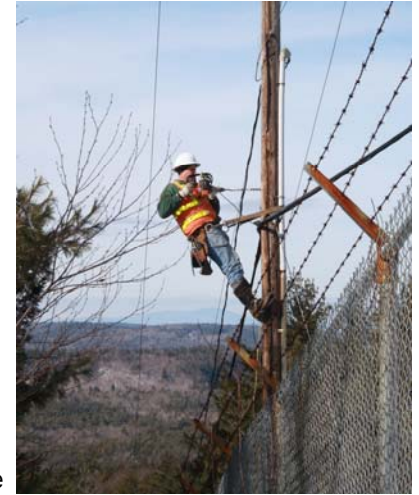
New Hampshire Optical Systems technician prepares one of 21,604 poles for fiber
