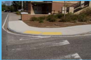
Curb Ramp with Brail Curb Warning
