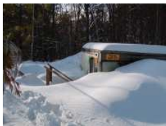
Water Treatment Building For Apartment Complex Pelham, NH
