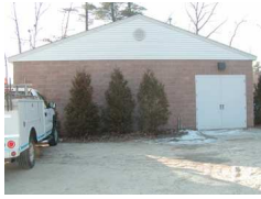
Water Treatment Building For Windham Public Water Windham, NH
