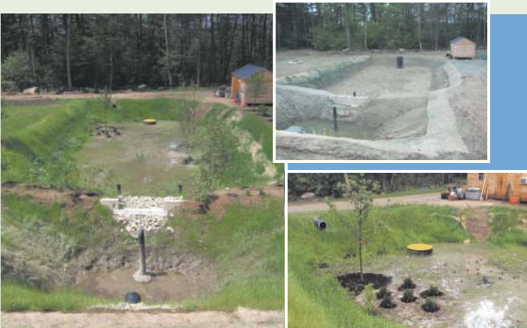
Hydroseeding and erosion control matting protect this system after installation [center]. Native species were planted along the installed system's [left] forebay and bioretention cell. Vegetation and appropriate soil media combine for effective water quality treatment [right].
