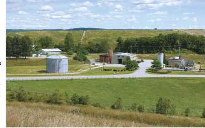
Waste Management's Turnkey Recycling and Environmental Enterprise Facility (also below) in Rochester, N.H.
